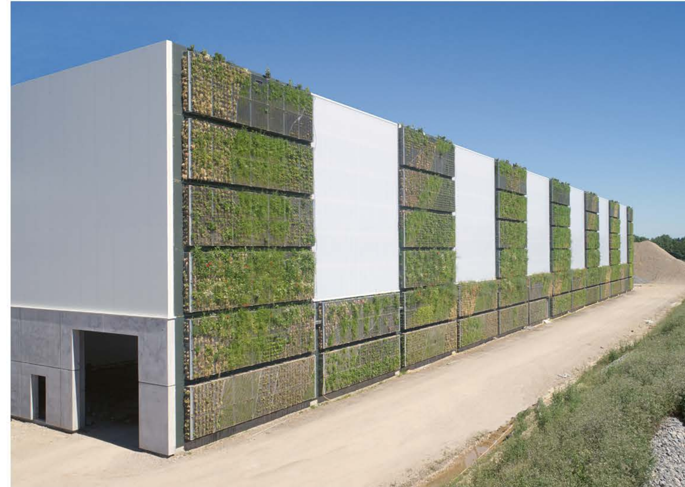
Werkshalle | Factory hall
