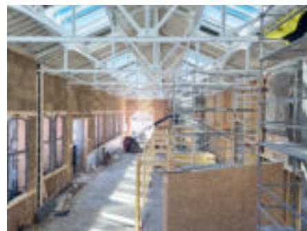
Dämmung aus Reisstroh. Insulation made of rice straw.
